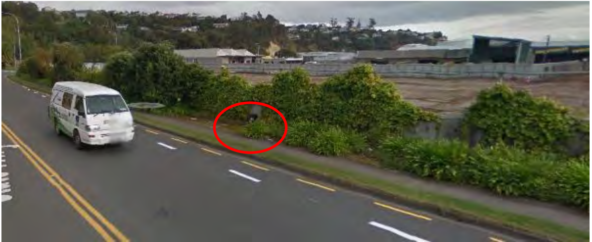
Figure 11: Port Nelson Log Yard Corner Wildman Avenue and QEII Drive, Showing Tilt Slab Wall and Power Junction Box.
