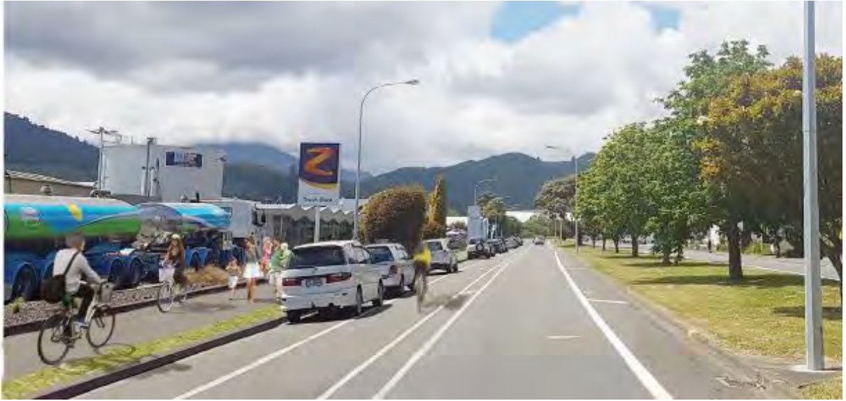
Figure 5: Option 3 Photo Simulation with On-road Facility as per Option 1 with Bi-directional Shared Path on the Seaward Berm
