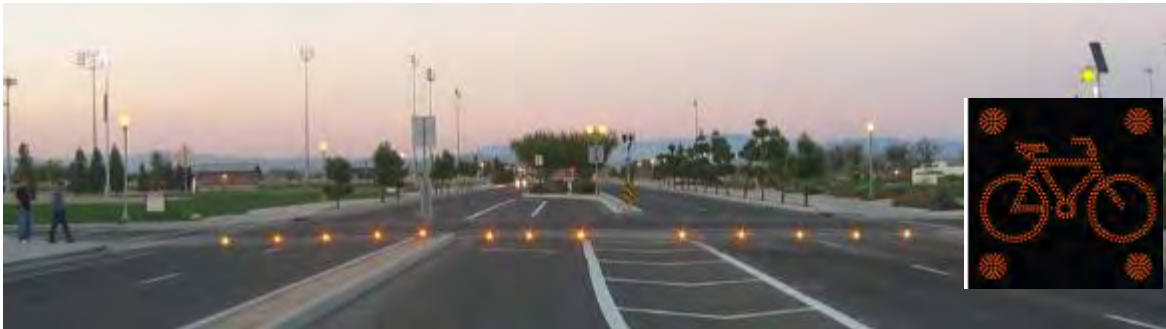
Figure 2: Examples of Electronic LED Smart Studs and Electronic Cycle Signs Proposed for Hay Street Intersection
