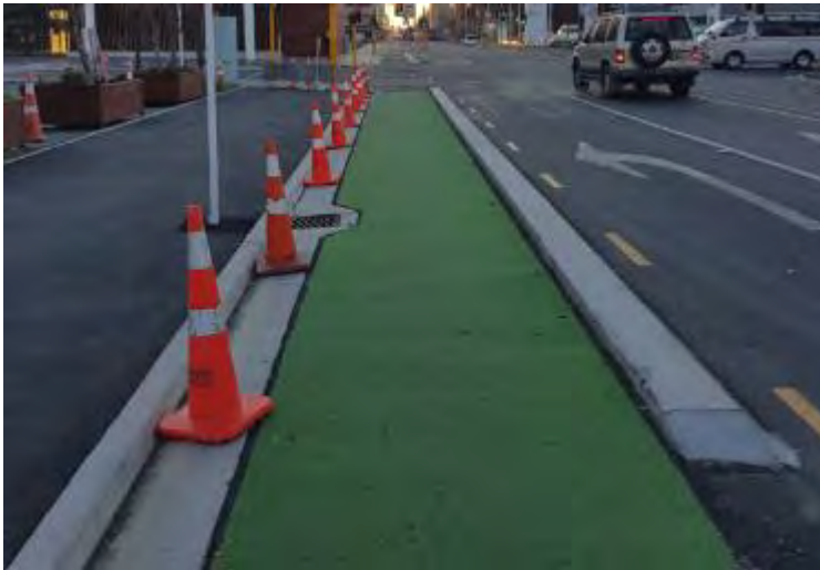
Photograph 2: Example of a mono directional separated cycle lane from Christchurch NZ
