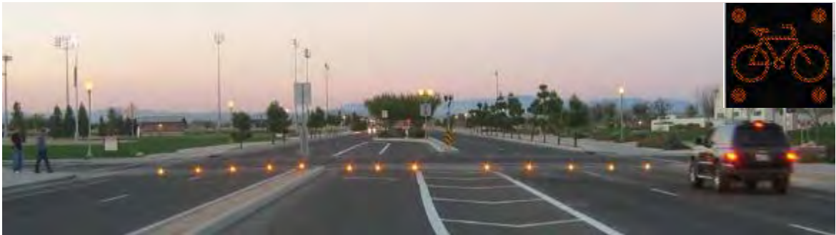
Figure 25: International Example of LED Smart Studs and Electronic Sign Used at a Crossing Point
