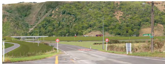
Figure 126 Indicative view down Poplar Ave to Expressway over bridge
