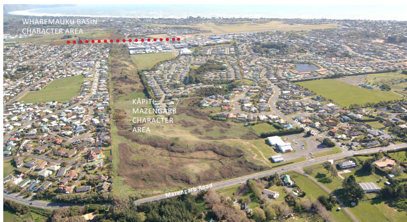
Figure 57 Mazengarb Road looking south
