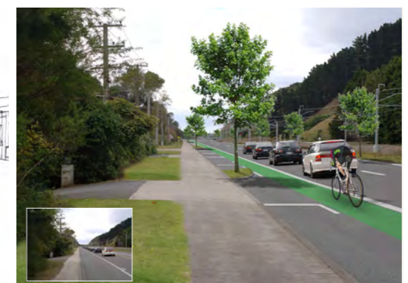
Figure 122 Photo simulation of SH1 at Raumati showing possible increased berm width, parking and cycle lane marked
