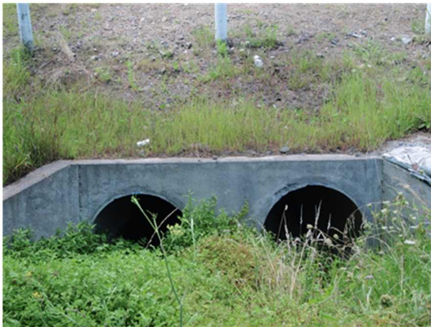
Photo 3 - Existing Hadfield Kowhai culverts under SH 1, with Mimulus sp covering waterway
