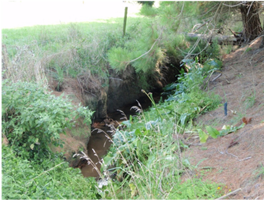
Photo 2 - Hadfield Kowhai Stream taken from SH 1 culvert
