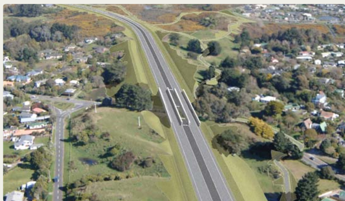
Indicative aerial view of the Raumati Road expressway bridge. The shared cycle/walk path can be seen on the right - before mitigation work.
