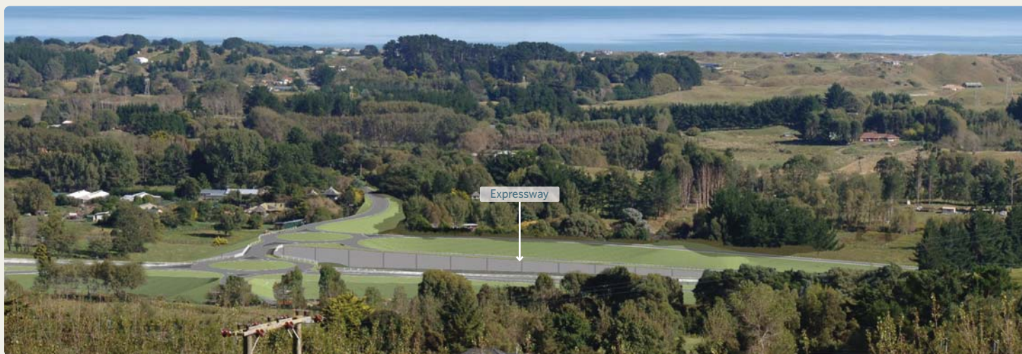
Indicative view of expressway from Hadfield Road area looking west - before mitigation work.
