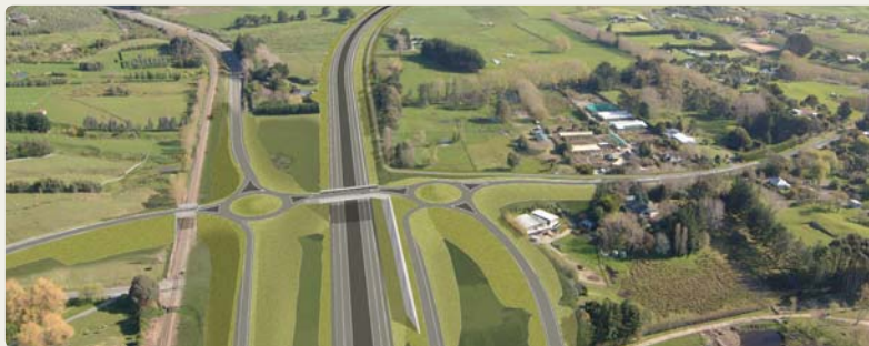
Indicative aerial view of the partial interchange at Peka Peka Road looking south. A new elevated crossing over the railway is provided for Hadfield Road - before mitigation work.
