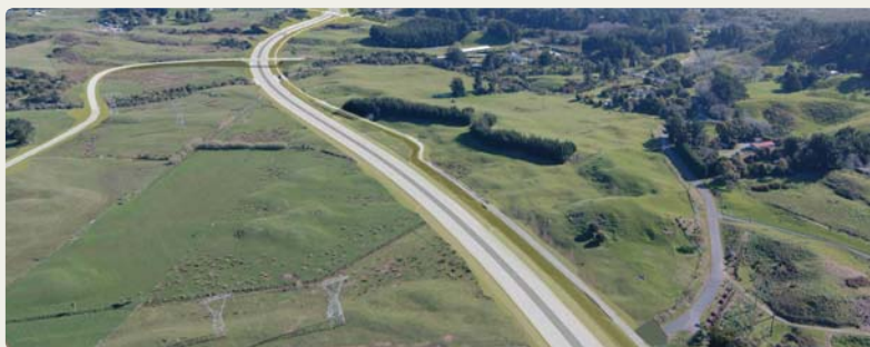
Indicative aerial view of the new connection overbridge looking south. Smithfield Road is closed - access to Nga Manu (in the top left corner of the image) will be from the new local road. The shared cycle/walk path can be seen on the west (right) side - before mitigation work.
