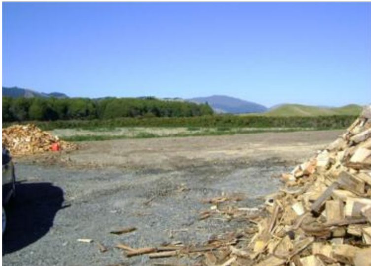
Figure 12: showing fill placement
