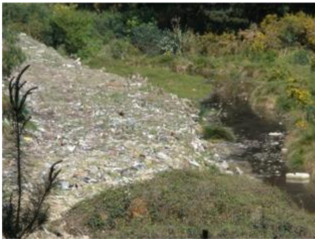
Figure 15: Otaihanga Landfill – Landfill Drain.
