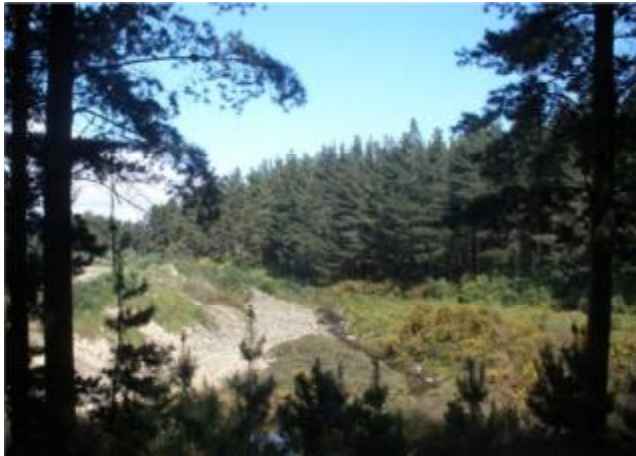
Figure 14: Otaihanga Landfill – toe of landfill, route to the right in the pine trees
