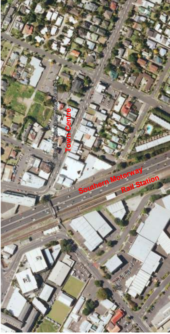
Left Aerial view of the Southern Motorway between Ellerslie Town Centre and Ellerslie Railway Station.
