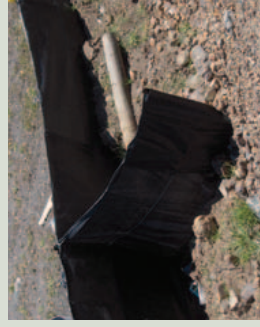
Picture: Silt fence return – minimum 1m upslope.
