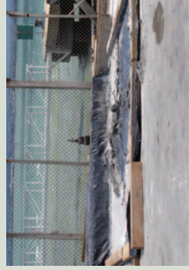
Picture: Timber-lined washout area.
