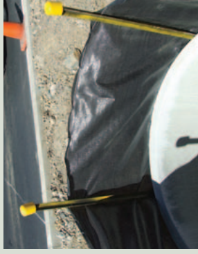
Completed Silt Fence protecting manhole.
