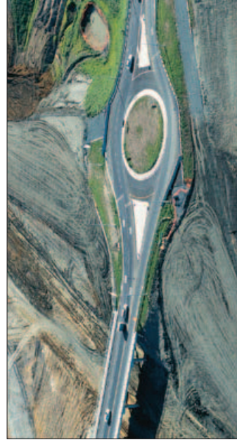
Orewa Interchange construction, ALPUFT B2 Northern Motorway Extension
