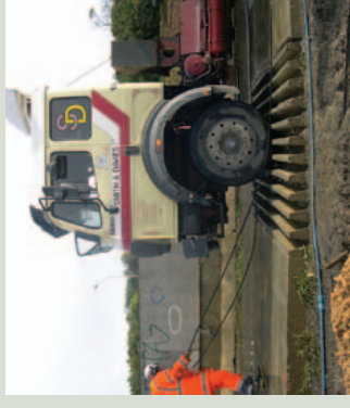
Picture: Wheel wash – concrete pad.
