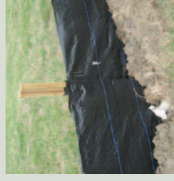
Correct silt fence joint.
