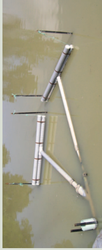
Picture: Sediment Retention Pond decant detail.
