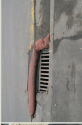
Maccaferri sand sock protecting a cesspit.
