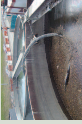
Picture: Settling tank.
