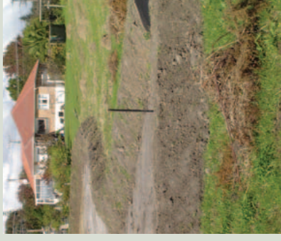
Picture: Diversion bund diverting clean water away from the construction area.
