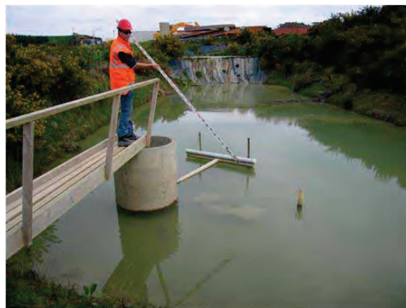
Undertaking Maintenance of a Sediment Retention Pond
