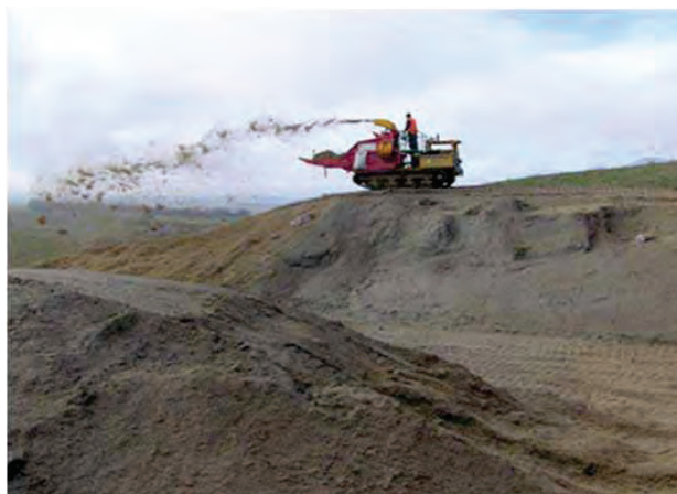
Erosion Control – Mulching
