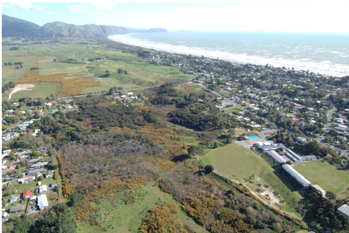
Photo 6.2: Sector 1 (Facing South)
