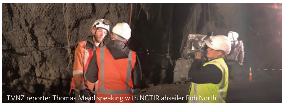
Once the first canopy post was installed, the remaining 13 followed closely after
