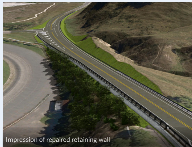
Damaged retaining wall above the racecourse
