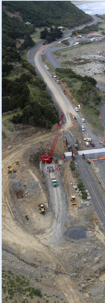
Jacob's Ladder temporary rail bridge removed
