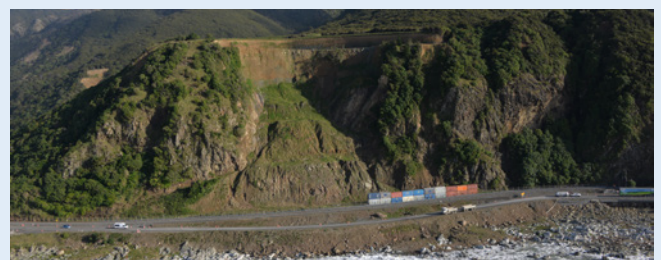
The hydroseeding on Site 8 at Waipapa Bay is proving successful as it's looking less like the site of a major slip and more like an integral part of the scenic coastal route.
