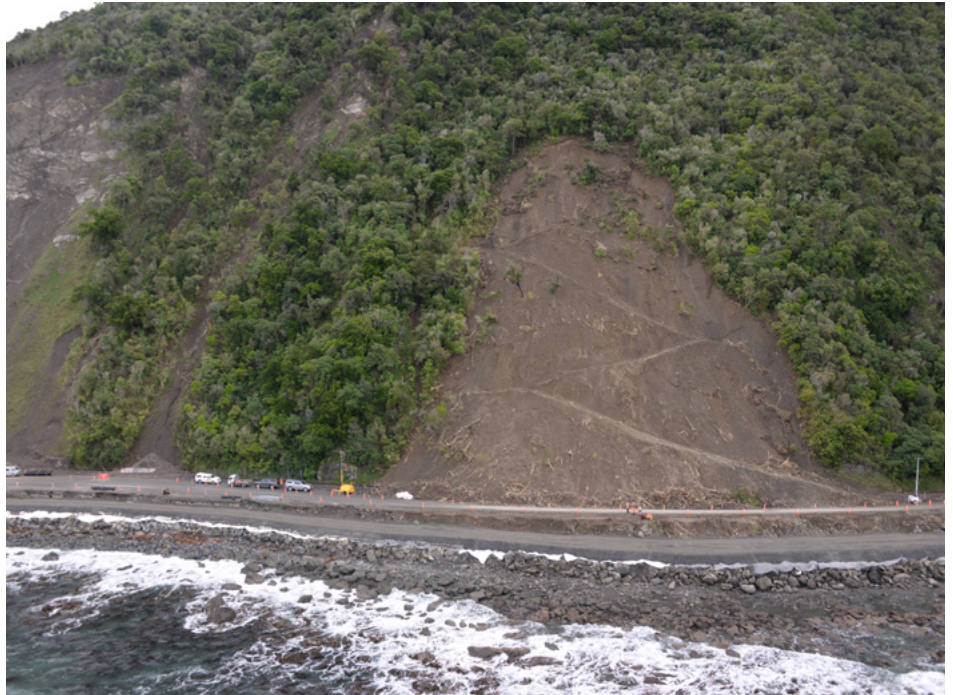
Slip 29A not long after ex-cyclones Debbie and Cook in 2017
