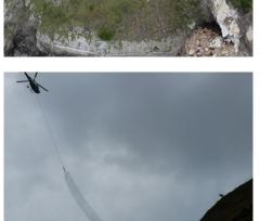
Safety and value for money are winning out at slip 23 south of Kaikōura as temporary rockfall protection is being made permanent. Mesh installed on the slip last year to get the road open safely before Christmas will remain as a permanent protection feature. At 45 metres high the mesh drapes over the cliff face having two functions:
