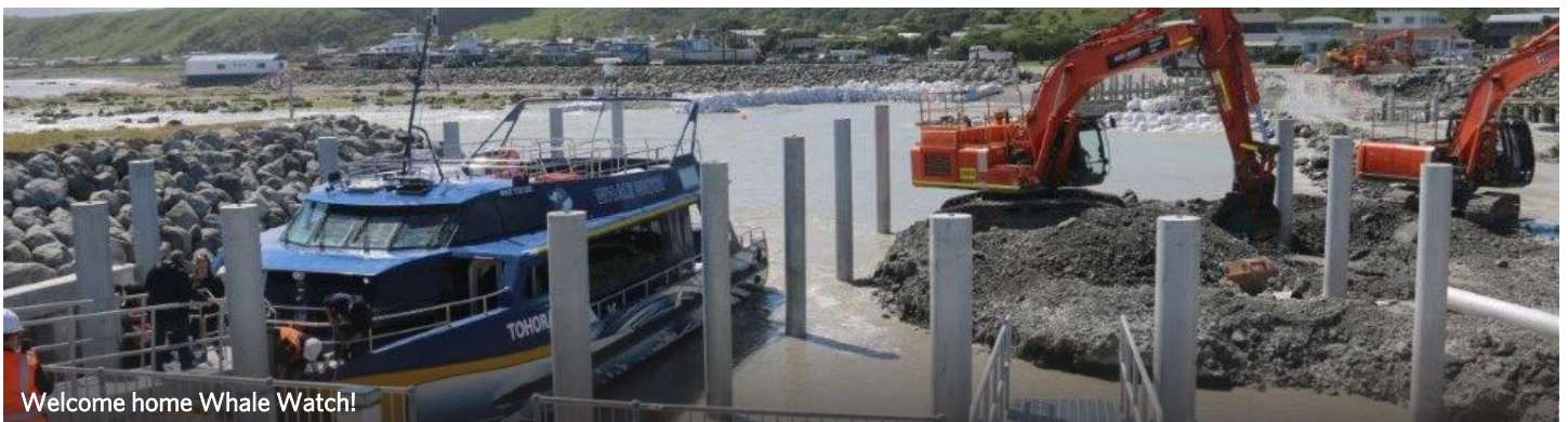
Getting the Kaikoura Marina ready for the first berth
