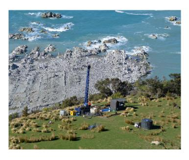
hill slope from the top of the slip, as well as from platforms that have been built into the face by abseilers. Once the inclinometer tubing is installed, a device is lowered into the tube to measure movement of the slope. 'If we drill deep enough, we will go through the possible failure, in order to see what is happening at depth, and this is really what we are looking to do,' says Brendon.
