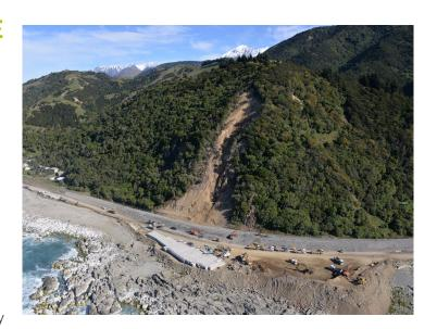
Last week about 7000 cubic metres of unstable rock and debris was removed during a helicopter sluicing and excavator exercise. The rail embankment has now been widened, new ballast placed and the track moved across up to four metres. The next step involves the placement of concrete blocks to form a low wall and working platform up the slope to allow the installation of the permanent rockfall protection structure.
