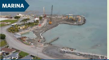
The Kaikoura marina was badly damaged during the earthquake when the seabed rose by up to two metres. It is on track to reopen in November 2017. The sea channel and harbour floor have been dredged back to their original depth and new retaining walls are being built along the promenade and rock groyne walls. A new Dolphin Encounter jetty and tender (small boats that ferry cruise passengers to shore) jetty are also being built.
