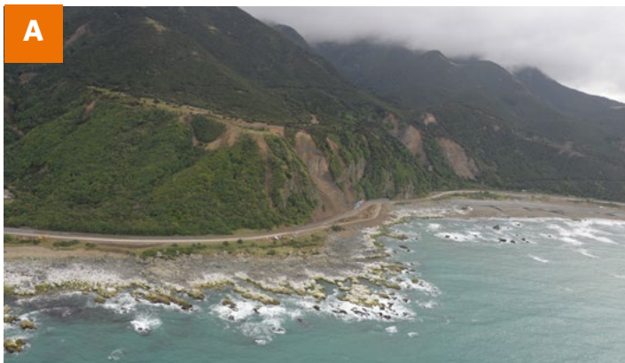
Looking north towards Site 8 you can see that much of the material has been cleared.
