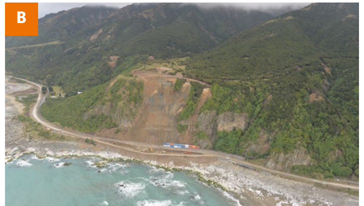
Looking face on to the slip face the bench and the container wall can be clearly seen.
