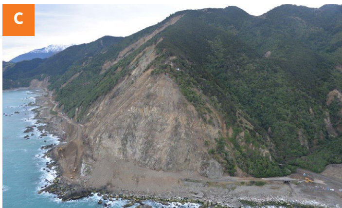
Photo showing the north side of Ohau Point and the extensive work done to clear the slips. The abseiler's base can be seen at the top of the hill.
