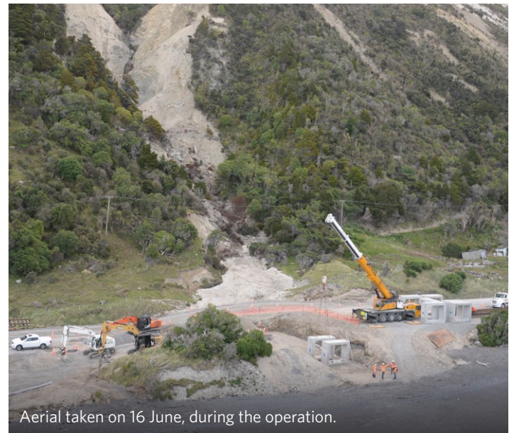
Off loading each unit, measuring 3m by 2.5m and weighing 17 tonnes each.
