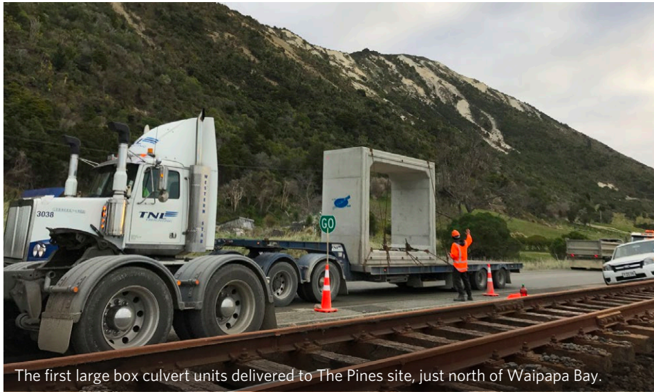
Off loading each unit, measuring 3m by 2.5m and weighing 17 tonnes each.
