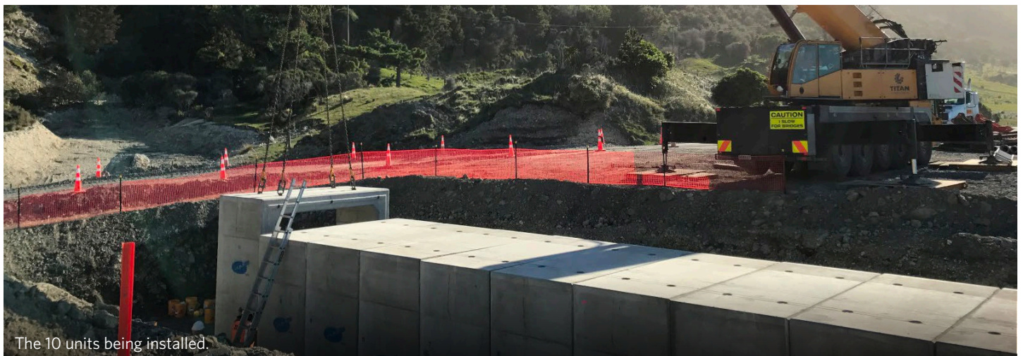
Installing the first unit within Mounseys Creek at The Pines. A total of 10 units were installed across the KiwiRail corridor.
