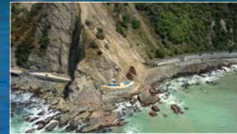
E Parititahi Twin Tunnels (Slips 14-20)
