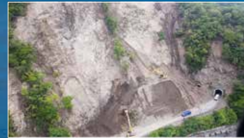
A Raramai Twin Tunnels (Slips 31-32)
