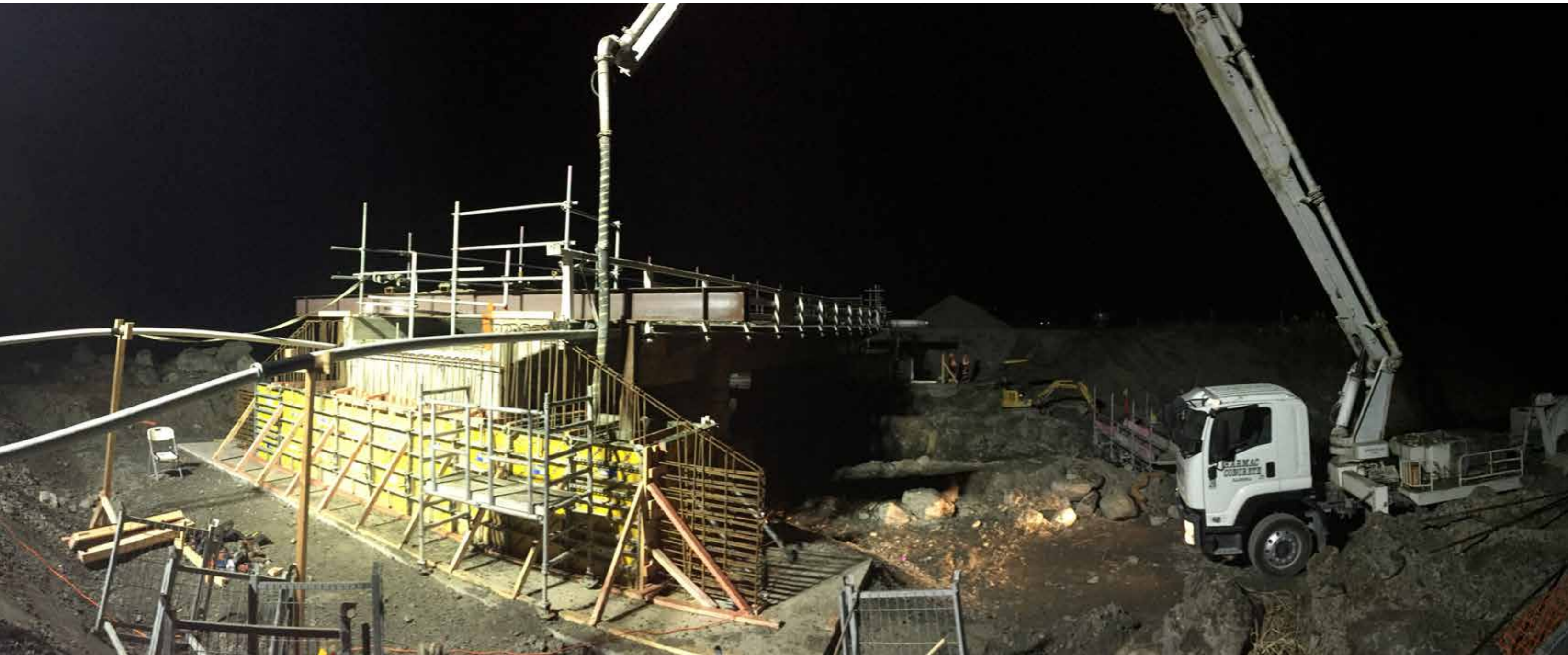
Response to Rebuild
