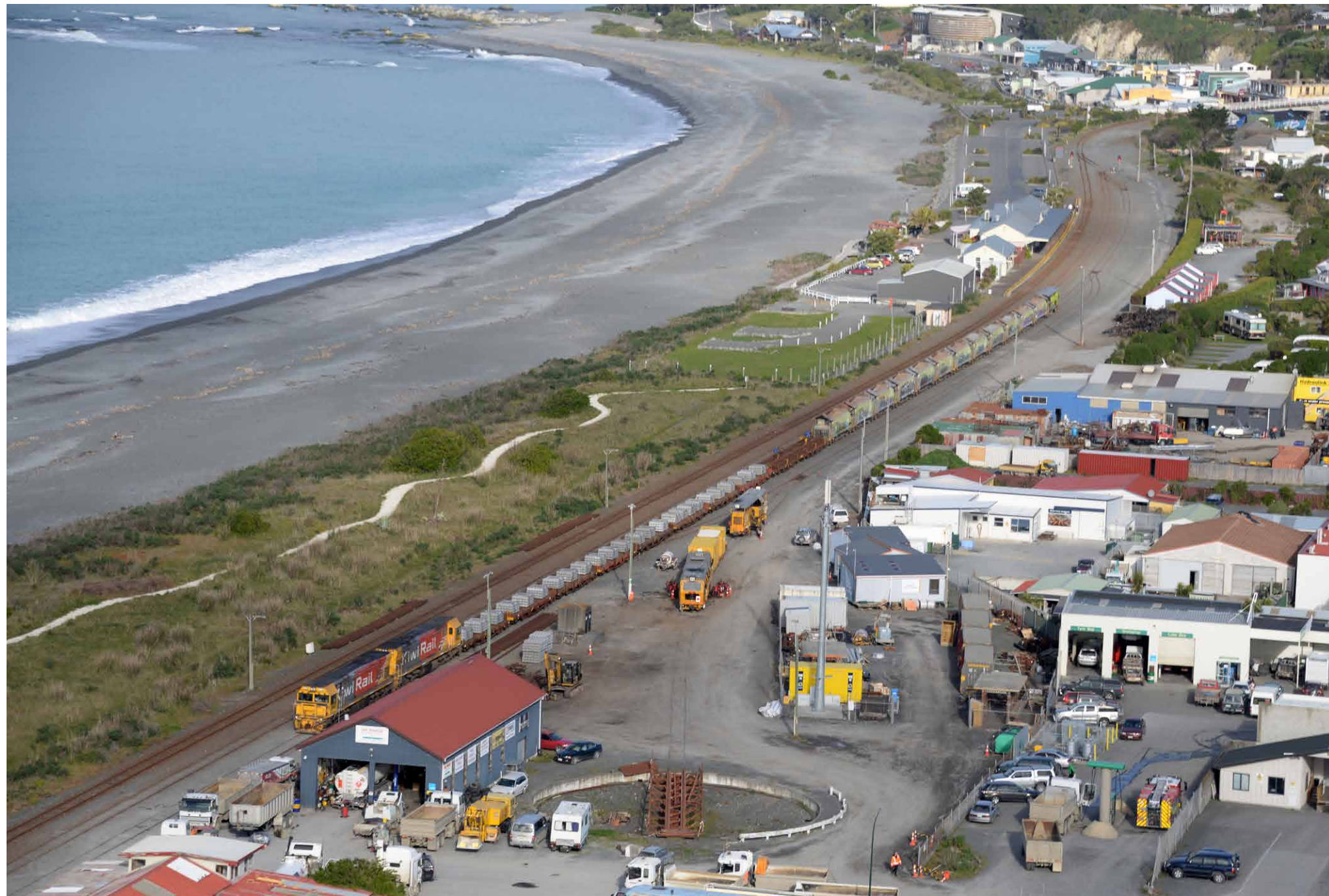
Response to Rebuild
