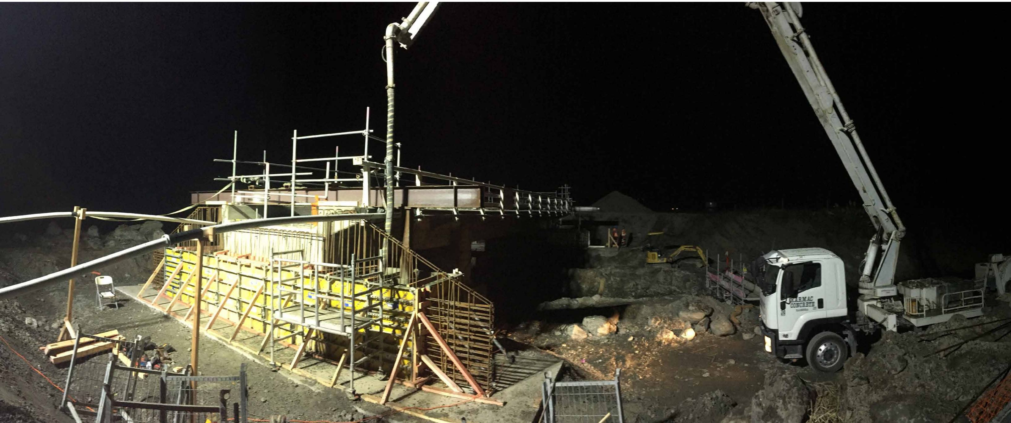
Response to Rebuild
