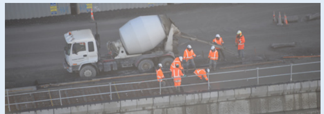
Crews are pouring concrete for the shared path at Ōhau Point north of Kaikōura – this will also act as the capping beam for the seawall. This is the location of one of the massive slips that cut off Kaikōura from northern access to State Highway 1 last year.
