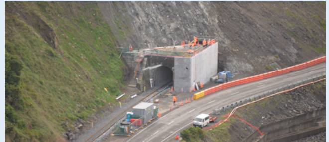
Tunnel 13 just south of the Kahutara Bridge is being transformed by the hard work of the tunnel crews involved.
