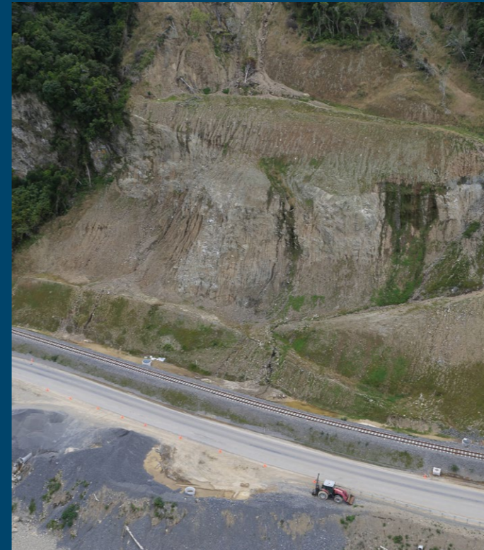
Earthquake slips at site 4 and site 8 were cleared last year and the slopes were scaled back to reduce risk of further slips. Benches were cut into them and seeds were sprayed at Slip 4, all of these factors stabilised these slopes which performed as expected in the weather.
