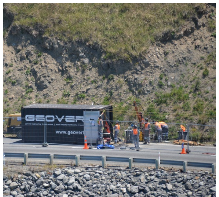
Crews are back on the road sharing it with travellers
