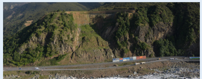
The hydroseeding on Site 8 at Waipapa Bay is proving successful as it's looking less like the site of a major slip and more like an integral part of the scenic coastal route.
