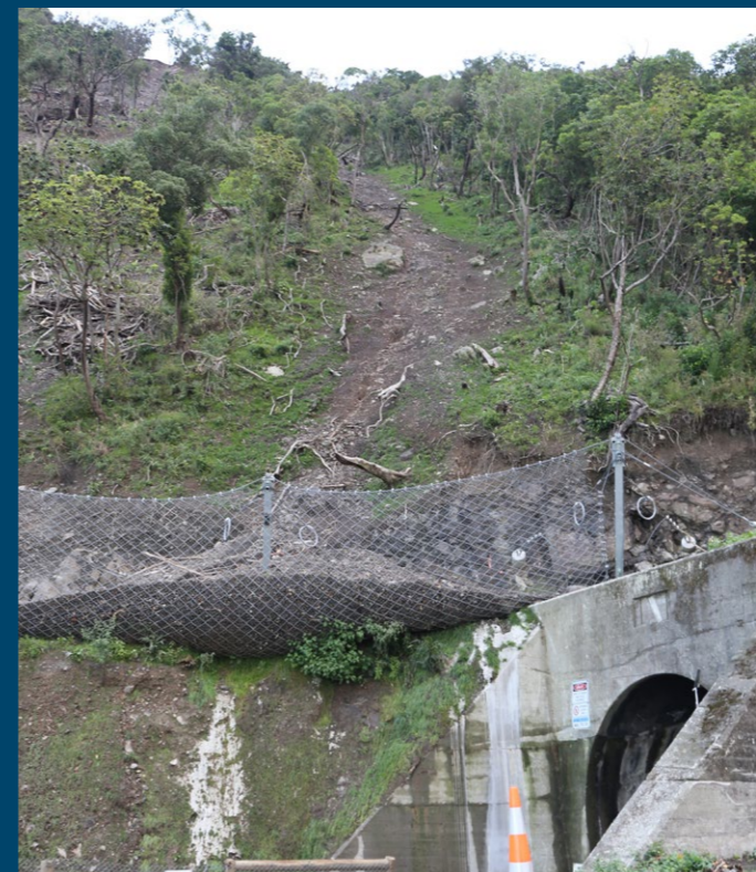
Adjacent to Raramai Tunnels, south of Kaikōura the rockfall fences have collected material, keeping it from falling on the rail below. The material collected has been emptied safely.
