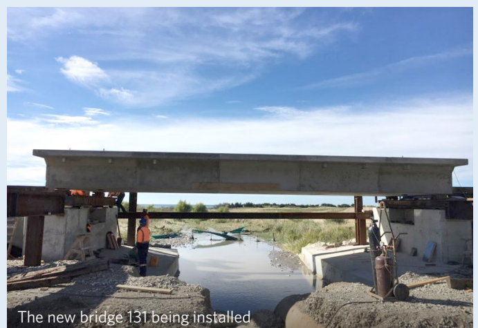
The temporary 'ugly bridge'
