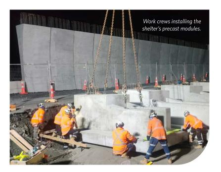
The shelter includes 165 pre-cast concrete modules made off-site then transported to the tunnel for assembly. These played a major part in the fast, safe, and efficient completion of the new shelter that replaces the previous 86-year-old avalanche shelter.
