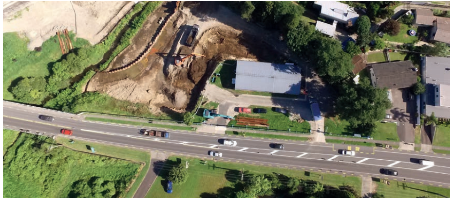
Asbestos area near the Baden Powell Hall.
