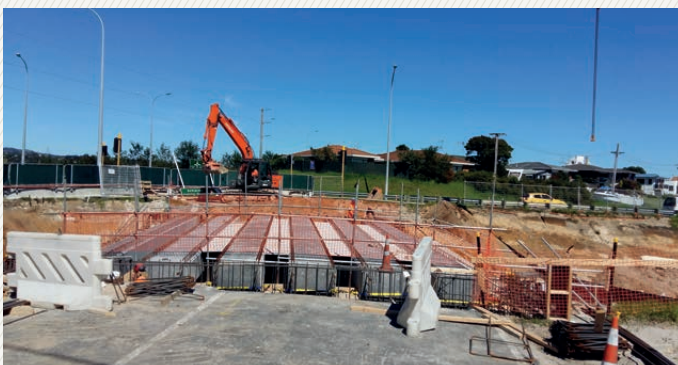
Image 1 and 2: Installation of bridge beams on western side of underpass
