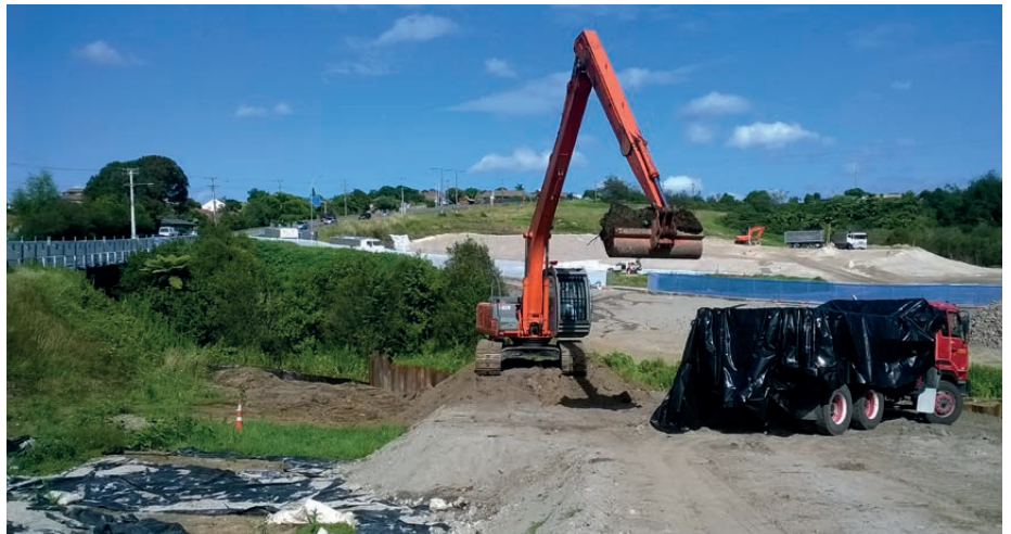
Asbestos removal underway. The material was loaded into fully lined trucks.
