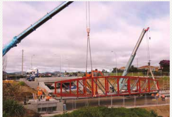
Two cranes lifted the 34 tonne steel bridge into place
