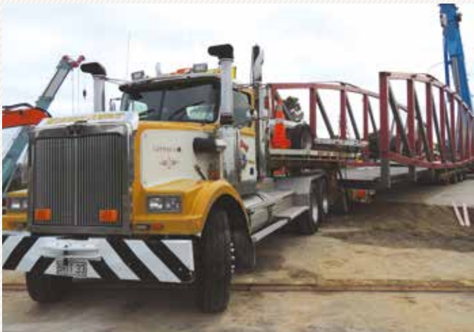
The steel bridge was delivered by truck from Napier
