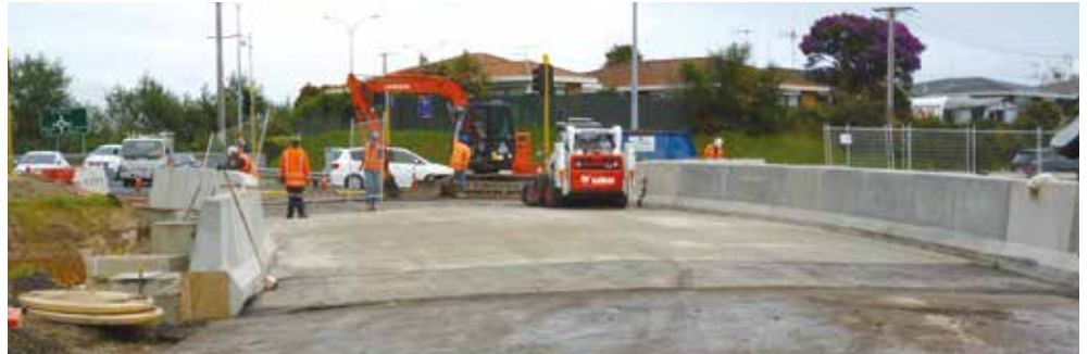
Maungatapu roundabout bridge one nearly completed
