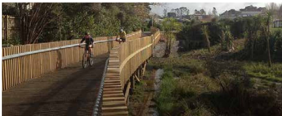
Elevated shared path suitable for sensitive ecological areas
