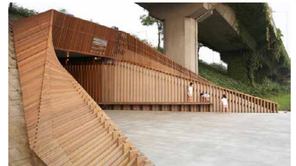
'Landing' the replacement pedestrian / cycle bridge over EWL to tie in with the existing underpass beneath MHX should create as open, clear and inviting an approach as possible
