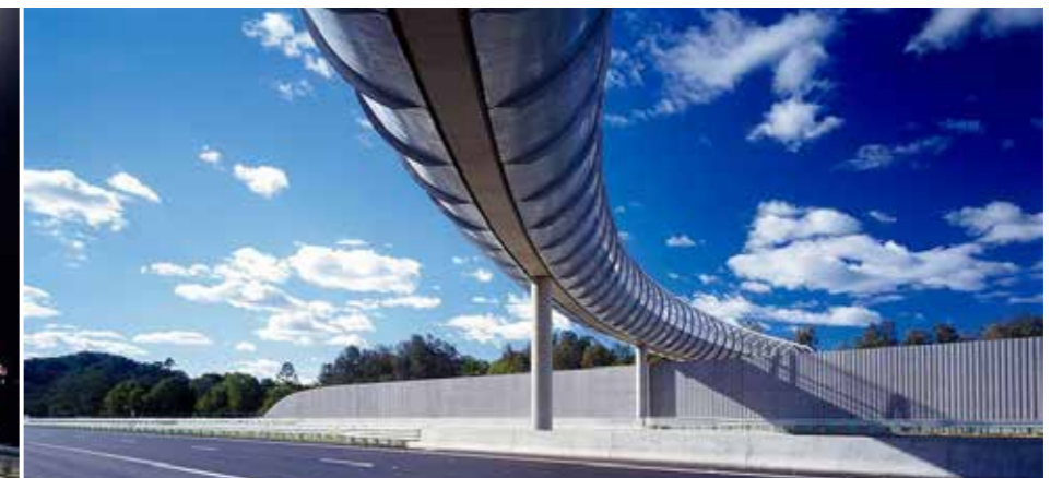
This shared path bridge (Pacific Highway NSW Australia) is a guiding precedent for the Alfred Street pedestrian / cycle bridge in its sinuous form, the materials palette, how it touches the ground lightly, integrates lighting with structure, and combines accessibility with simplicity
