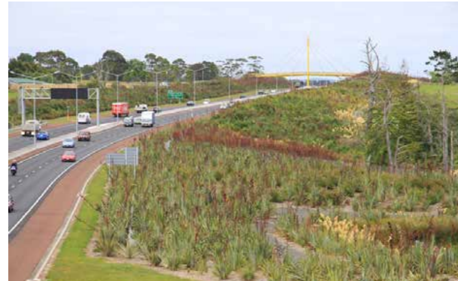
Hobsonville, Auckland - fill slopes shaped back into the contours
