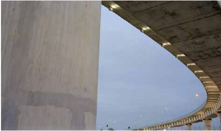
Westlink Interchange - elegant, simple curves create a sense of lightness
