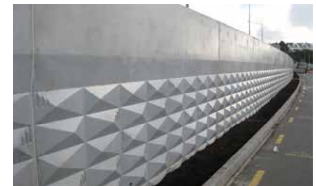
Westhaven Drive, Auckland - texture scaled to local road environment
