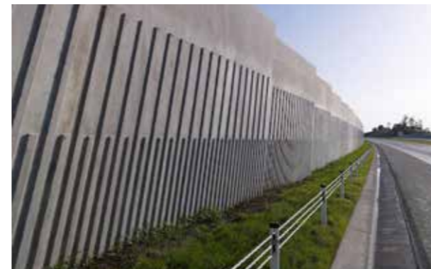
Pacific Highway, NSW - heavier patterning at the base grounds the wall in the landscape
