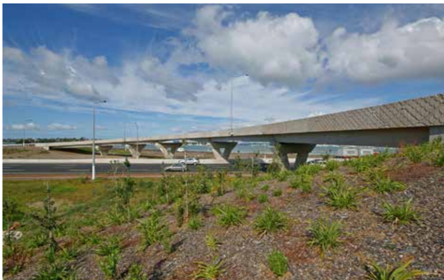
Open abutments integrated with the landform, and a unified appearance given by the parapet texture which relates to the pier form
