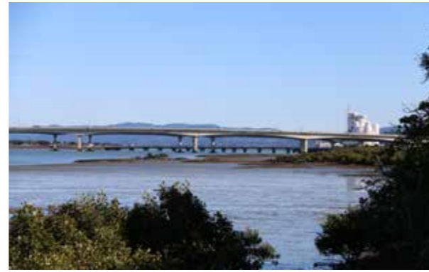
View towards Māngere Harbour Crossing (SH20)
