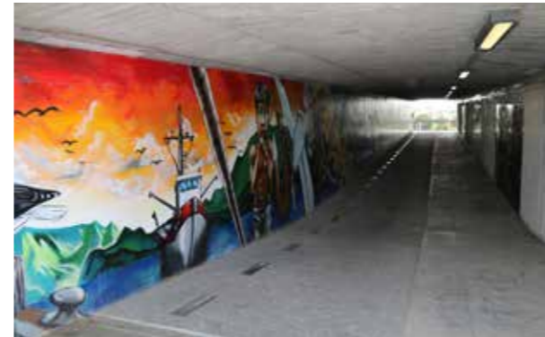
Lower Onehunga Mall underpass under SH20
