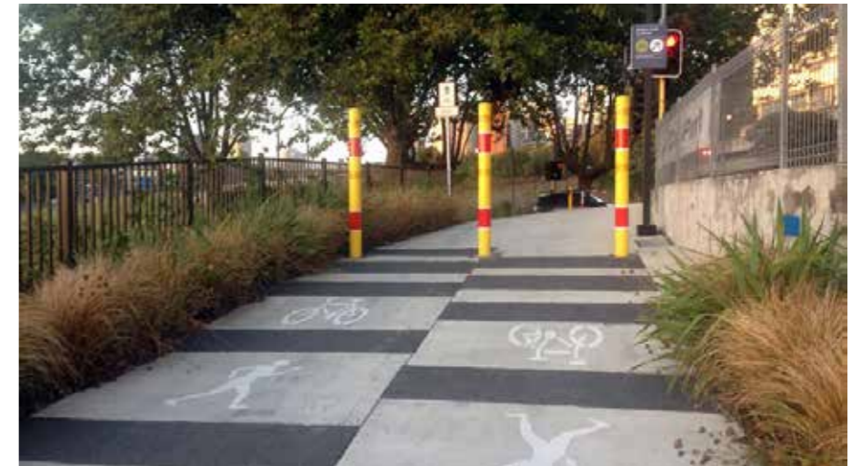
Clear delineation of direction of travel, transparent fences that allow overlooking of the shared path, and planting that softens the edge without blocking views or causing obstruction
