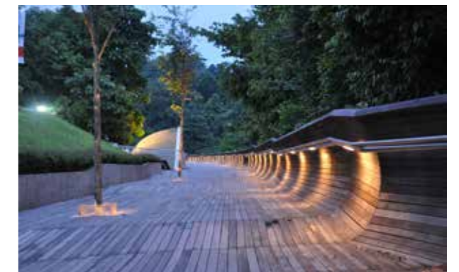
Integrated lighting with the balustrade creates a safe environment and a sleek appearance
