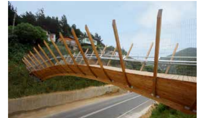
Light and transparent footbridge that integrates structure, screens and balustrading - a key feature is the gentle outward slope of the timber posts
