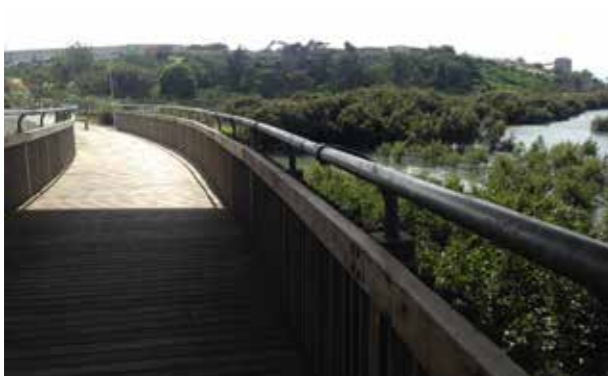
Boardwalk linking beneath SH20 to Waikaraka Shared Path
