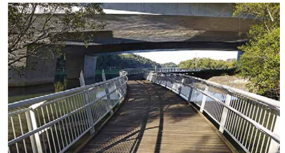
In recreating the shared path underneath the Manukau Harbour Crossing, provide an open and pleasant experience for path users
