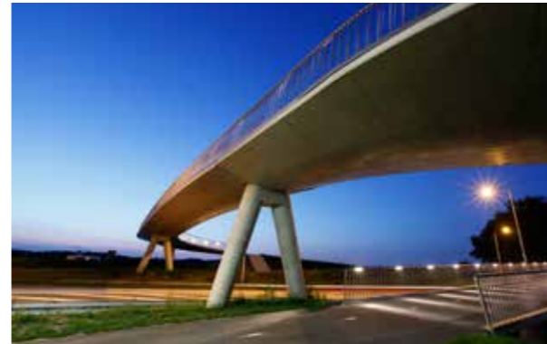
Heerhugowaard Cycle Bridge, Delft - touches the ground lightly with a sleek underside, slender deck and open balustrades, and sculptural piers
