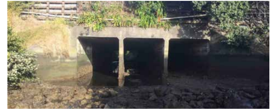
Ōtāhuhu Creek culverts under SH1
