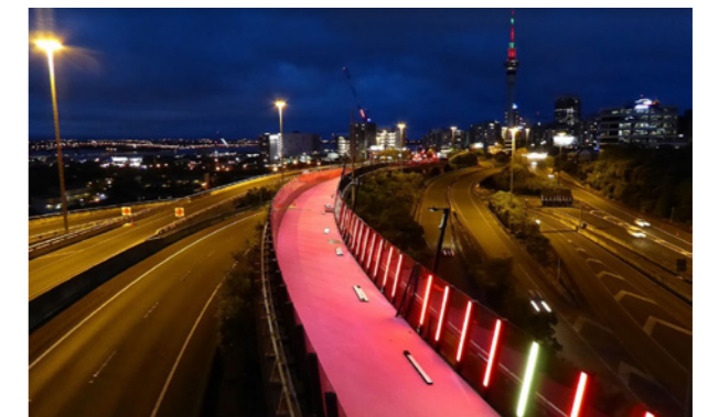
Auckland Lightpath - colour and lighting create a feature that highlights the ped/cycle path
