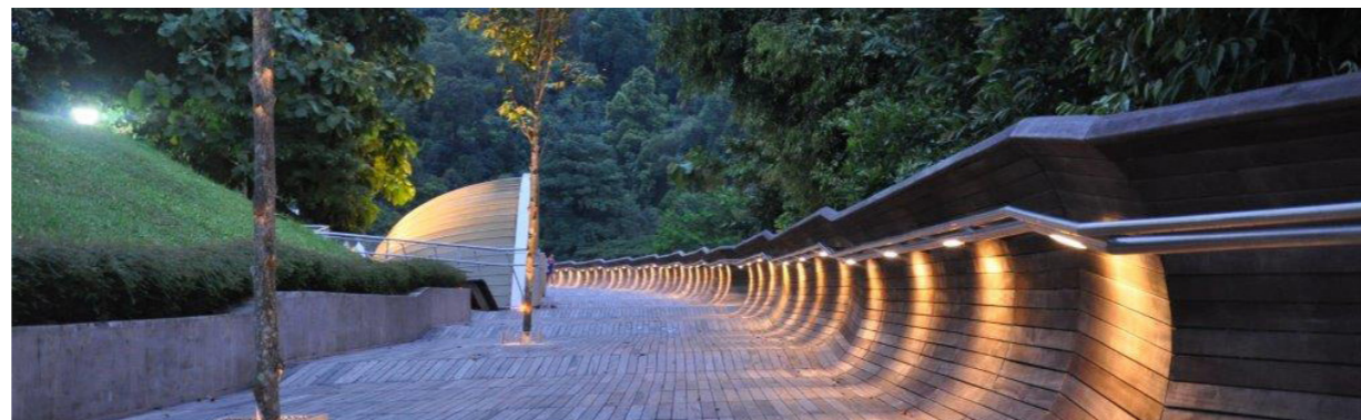
Henderson Waves, Singapore - good transition from structure to ground, simple, effective lighting integrated with handrail reinforces the form
