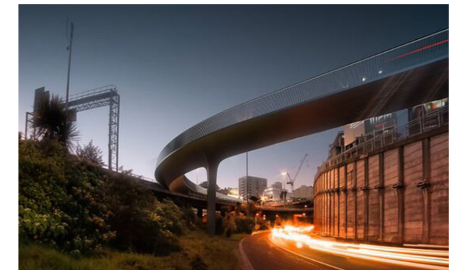
Auckland Lightpath - simple, elegant underside of structure with a single column
