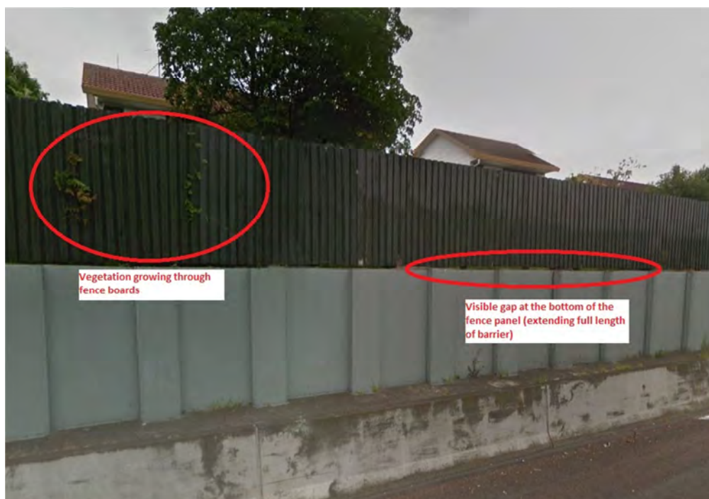
Figure 6-1: Barrier Ōtāhuhu northbound off-ramp
