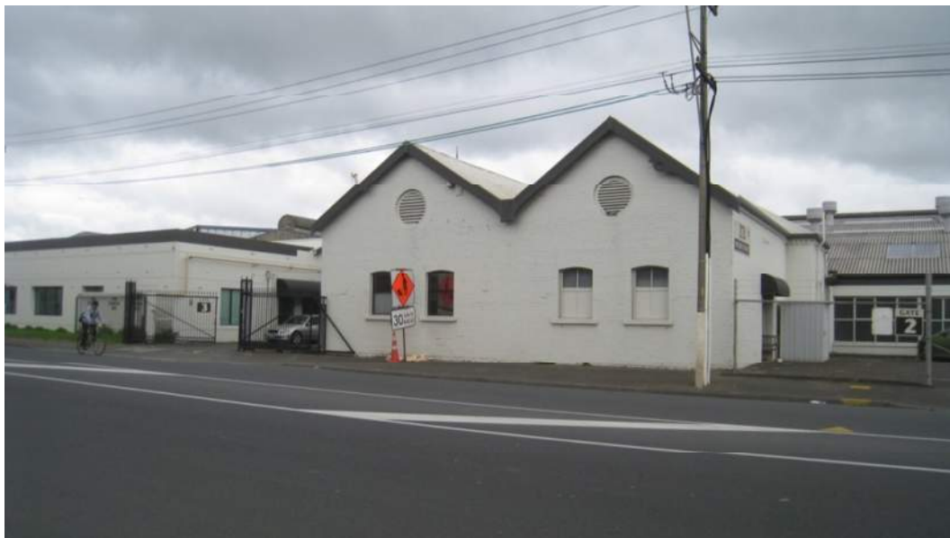
Figure 5-14: Onehunga Woollen Mills 273 Neilson Street. Photo Matthews & Matthews Architects Ltd, September 2016.
