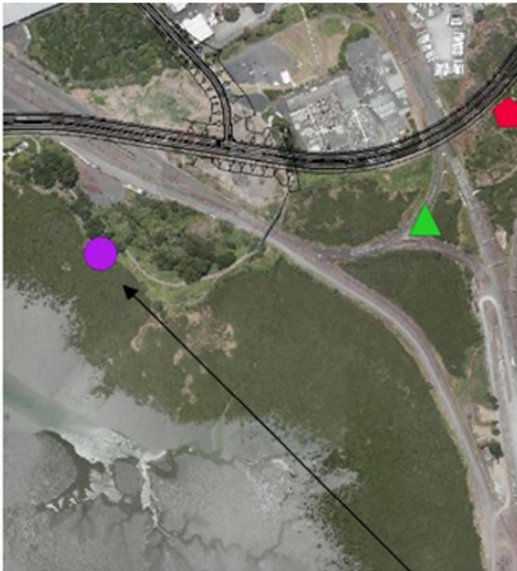
General Location of CHI ID 641 – Timber Sea Wall, Anns Creek Area
