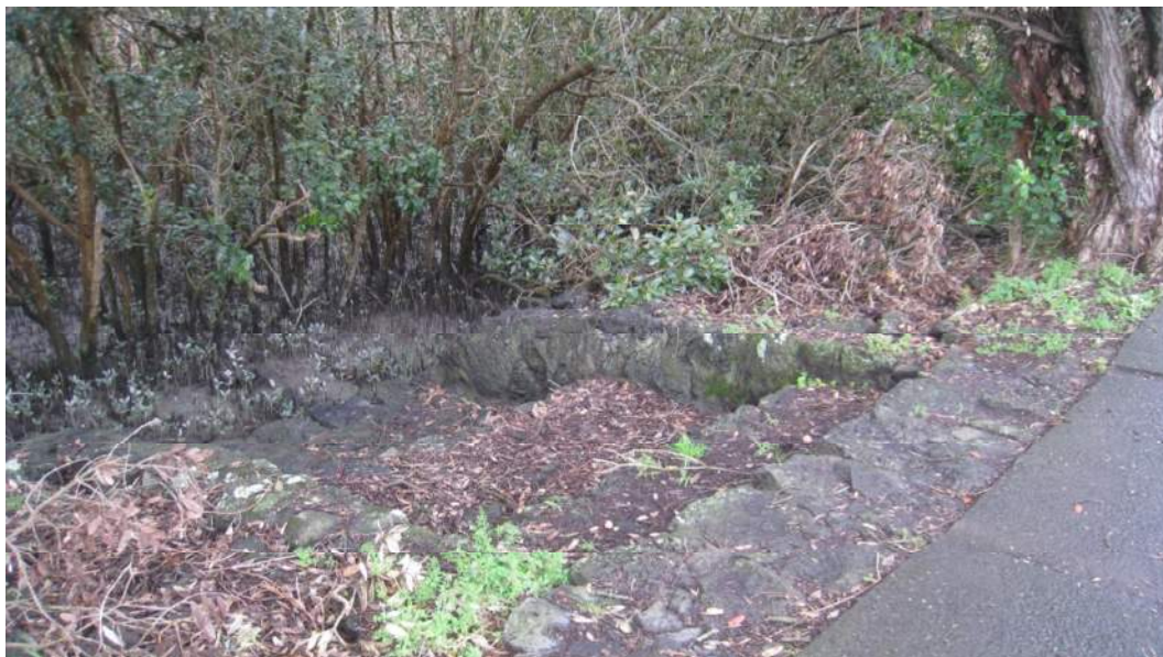
Figure 5-11: Stone stairs along coastal walkway. Photo Matthews & Matthews Architects Ltd, September 2016.
