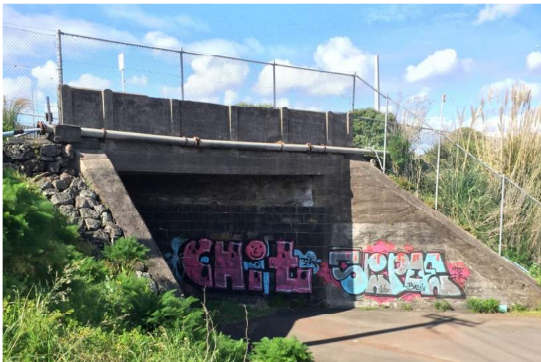
Figure 8-4: Rail bridge. Photo Matthews & Matthews Architects Ltd August 2016.
