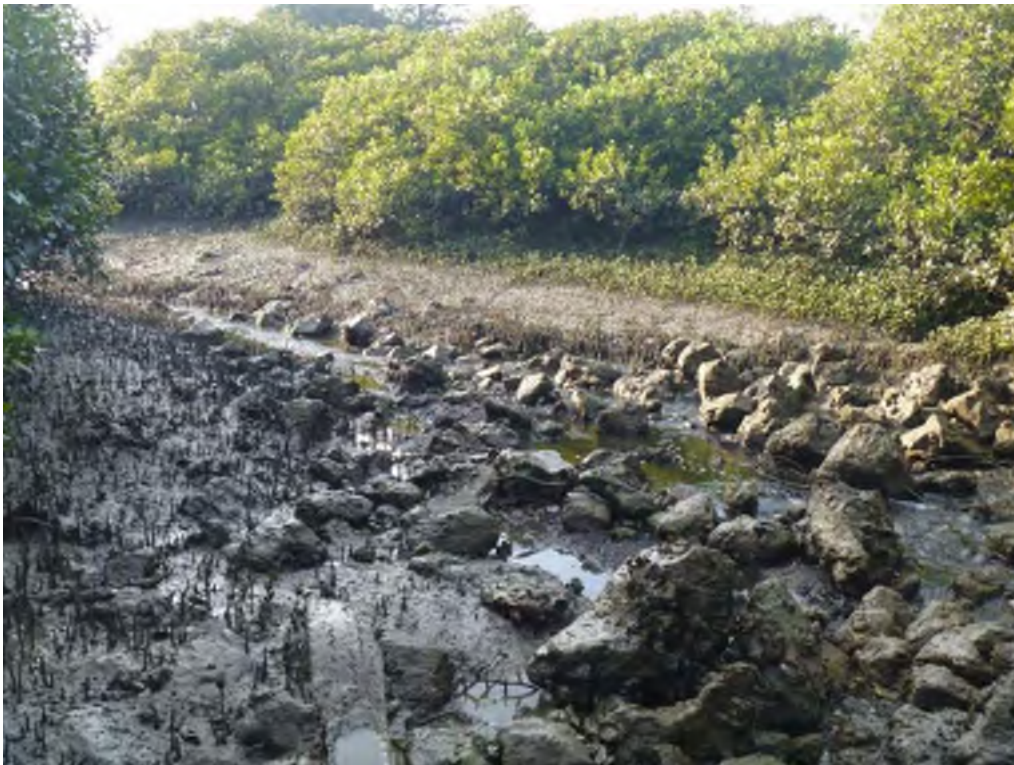
Downstream of box culverts in Otahuhu Creek.
