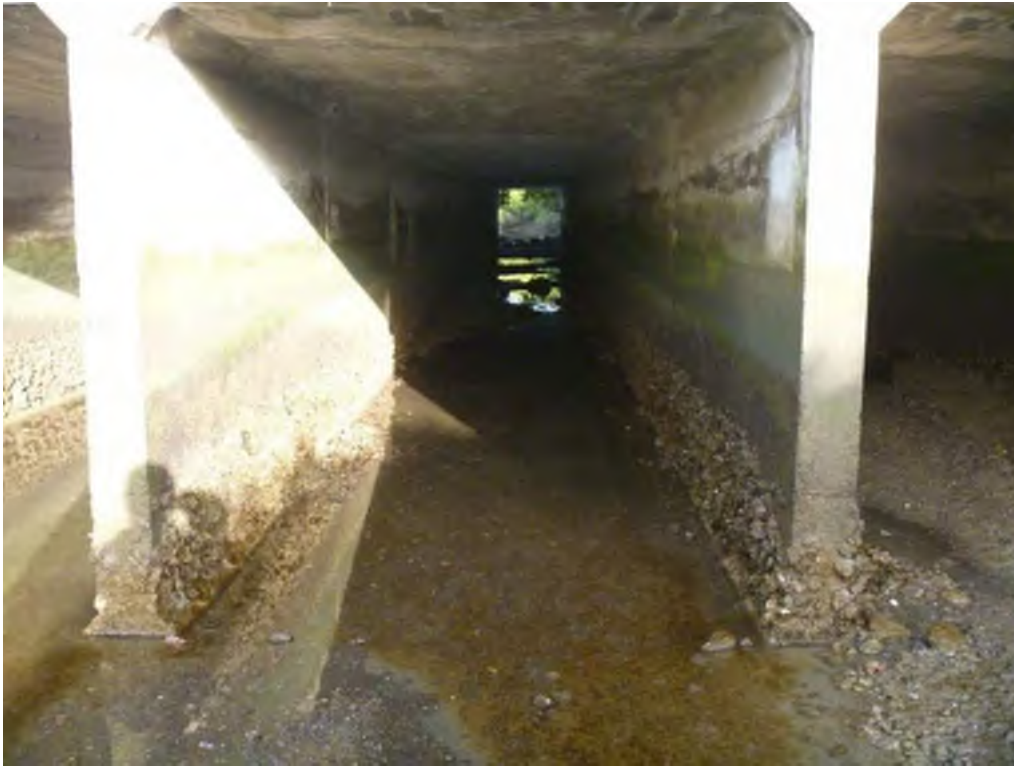
Box culverts under SH1 within Otahuhu Creek.
