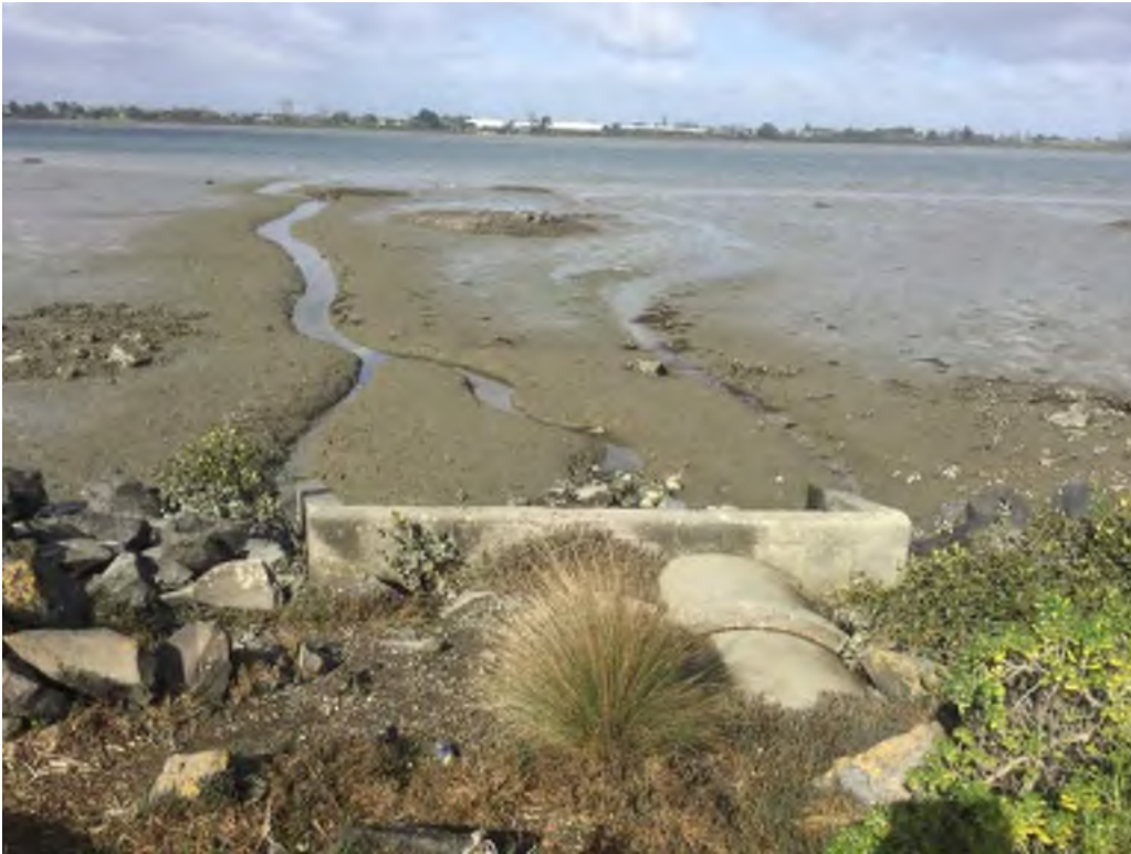
Miami Stream discharge point to CMA.
