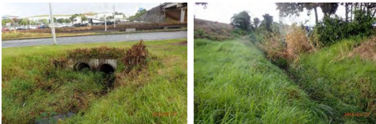
Plate 3-7: Clemow stream downstream culvert (left) and upstream reach (right).
