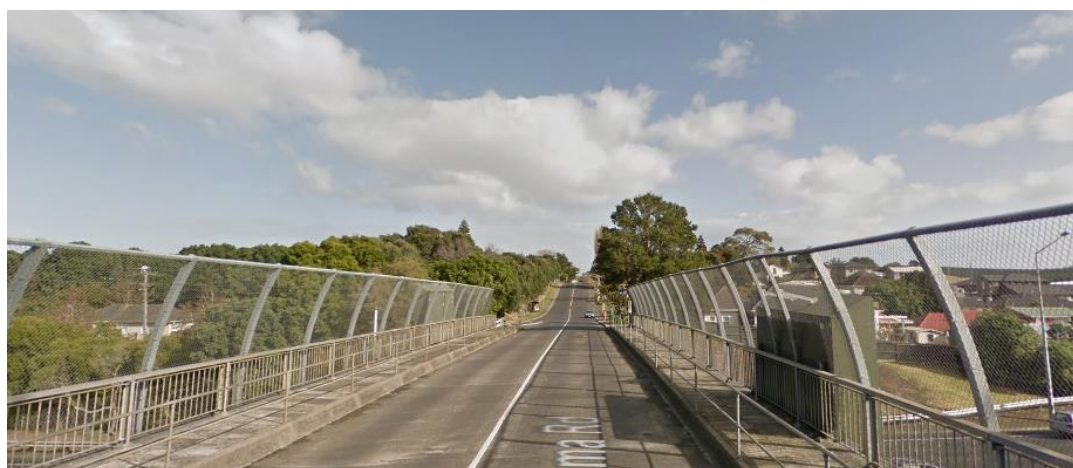
Figure 5-22: Panama Road Bridge
