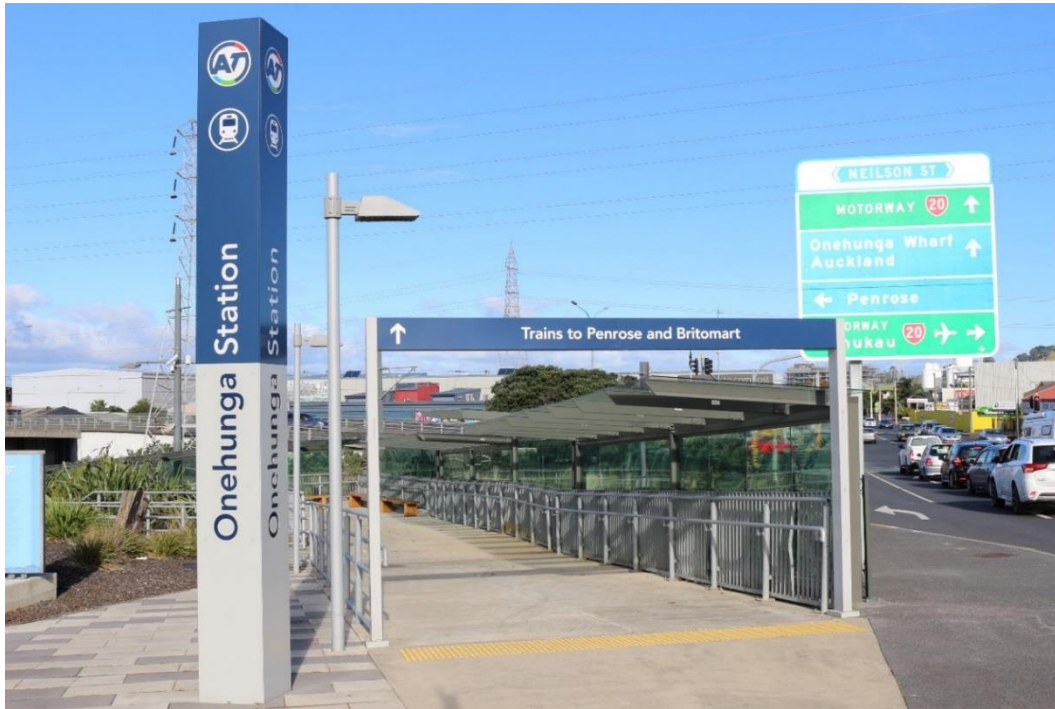
Figure 5-10: Entrance to Onehunga Train Station
