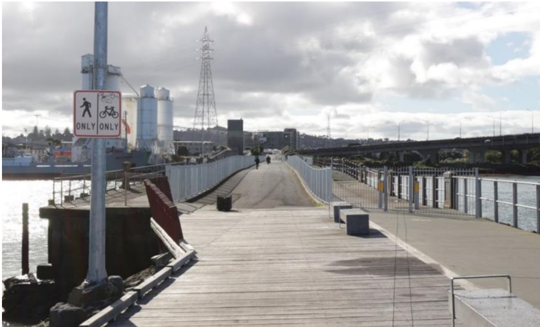
Figure 5-8: View of Old Māngere Bridge from the Māngere Bridge suburb end
