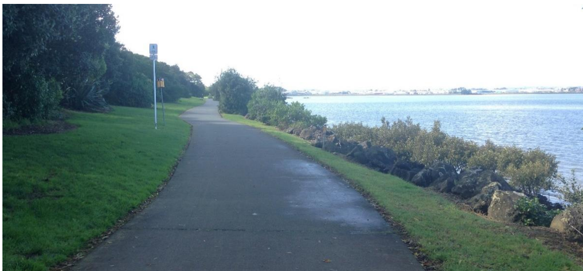
Figure 5-15: Manukau Foreshore East Walkway
