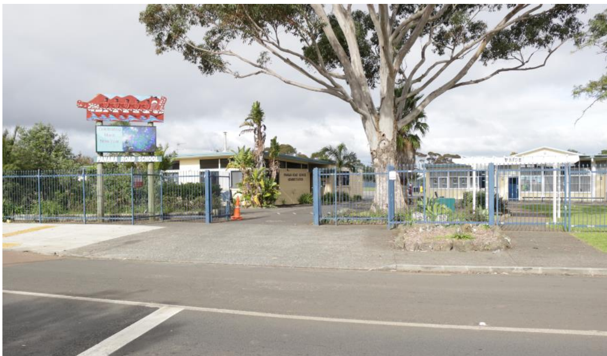
Figure 5-21: Panama Road School
