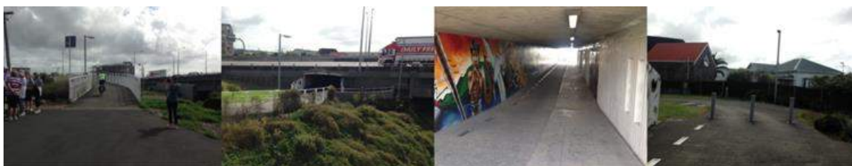
Figure 4-28: Onehunga Harbour Road Overbridge, underpass under SH20
