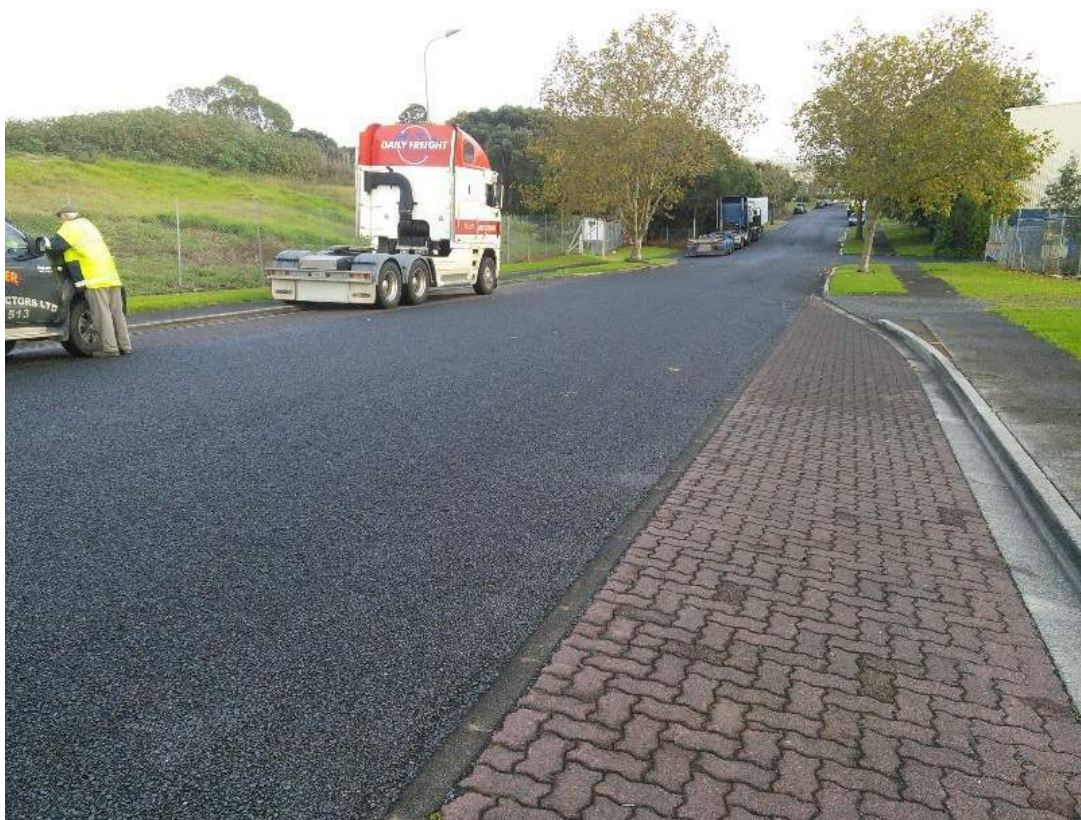
Figure 4-11: Hugo Johnston Drive Southern end (facing north).
