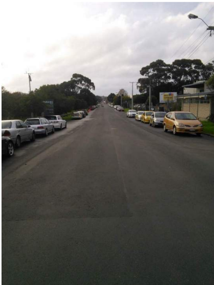
Figure 4-9: Captain Springs Road near entrance to Waikaraka Park looking North
