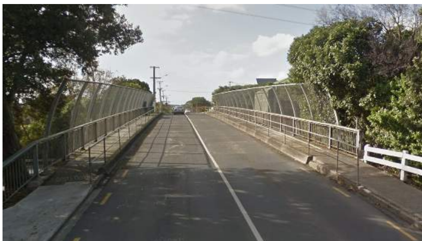
Figure 4-33: Panama Road Bridge
