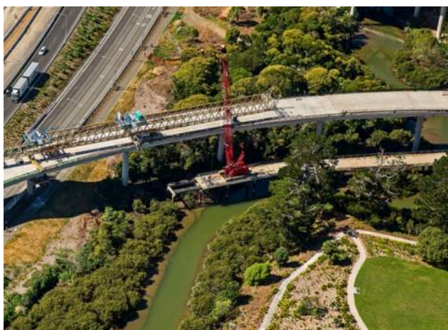
Figure 7-9: Temporary staging used for Great North Road Interchange (SH16)
