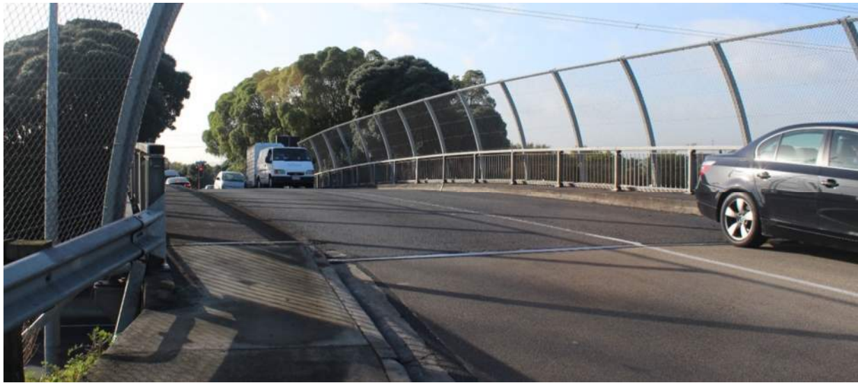
Figure 11-7: Princes Street overbridge (present day)
