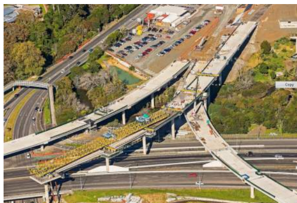
Figure 7-12: Construction of superstructure using a gantry
