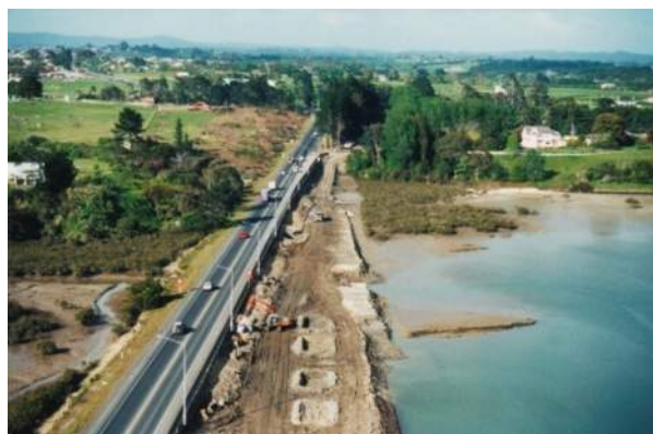
Figure 7-7: Reclamation using mudcrete for Upper Harbour Crossing (SH18, Greenhithe)
