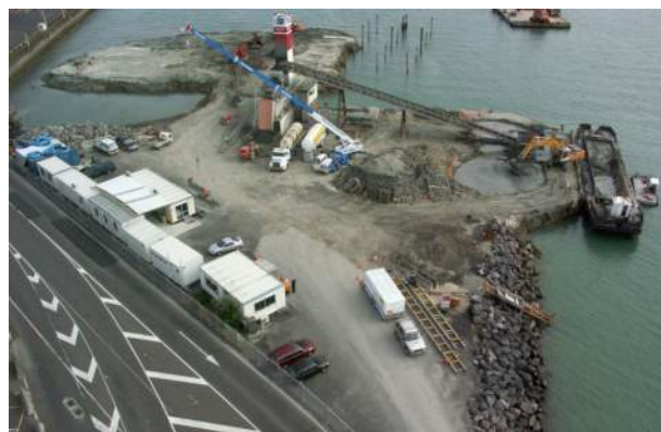
Figure 7-8: Reclamation using mudcrete at Fergusson Container Terminal
