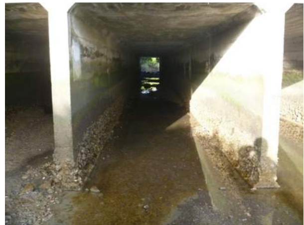
Figure 12-38: Ōtāhuhu Creek box culverts
