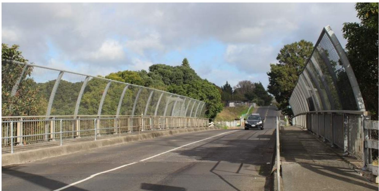
Figure 11-6: Panama Road Bridge (present day)
