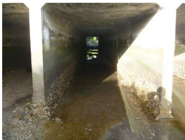
Figure 12-38: Ōtāhuhu Creek box culverts
