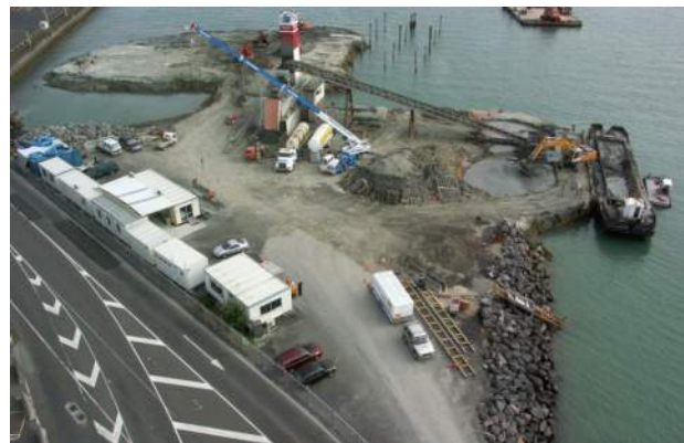
Figure 7-8: Reclamation using mudcrete at Fergusson Container Terminal
