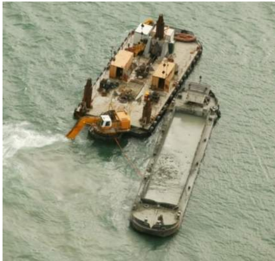
Figure 7-5: Typical dredging barge
