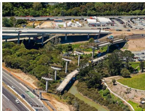
Figure 7-10: Construction of the substructure at Great North Road Interchange (SH16)
