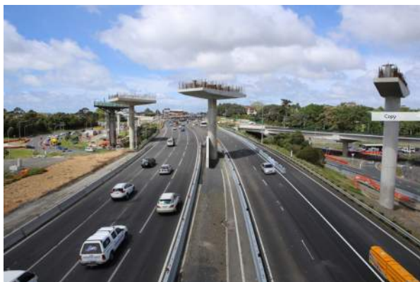
Figure 7-11: Ramp columns
