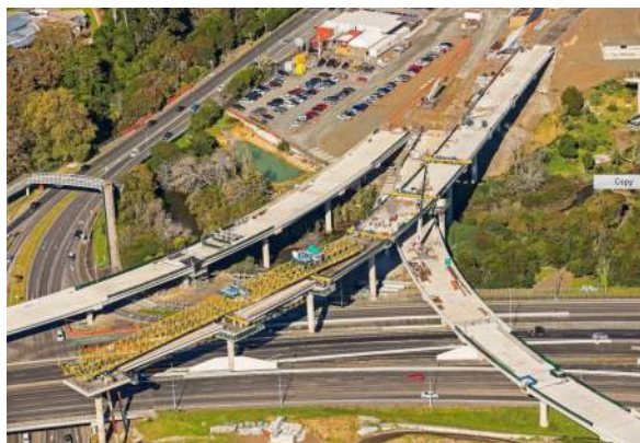
Figure 7-12: Construction of superstructure using a gantry
