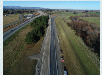
Widening of SH1 between the Waimakariri Bridge and the CNC motorway.
