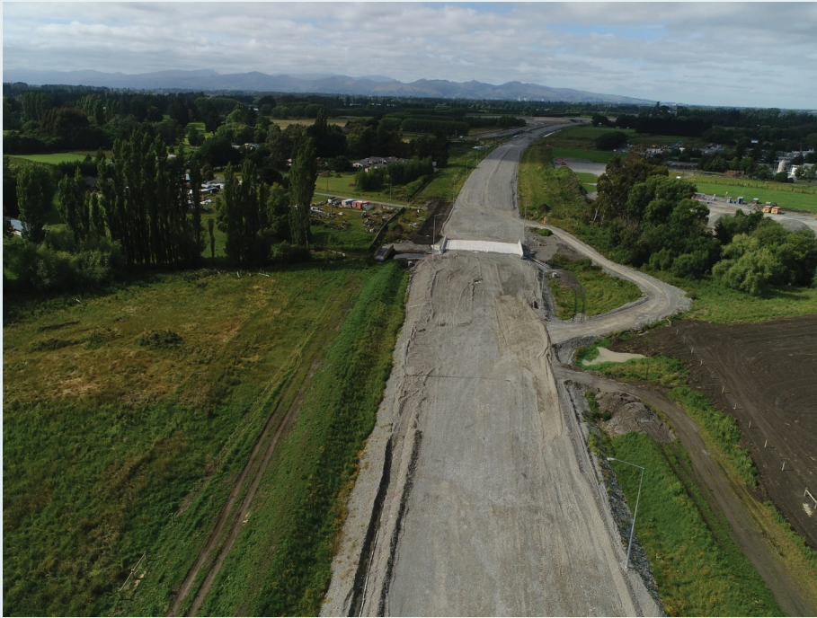
We have completed the Kā Pūtahi creek bridge.
