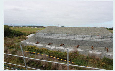
Styx River bridge abutment with surcharge layer of gravel.
