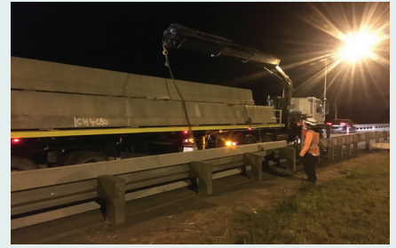
Safety barrier installation at night.
