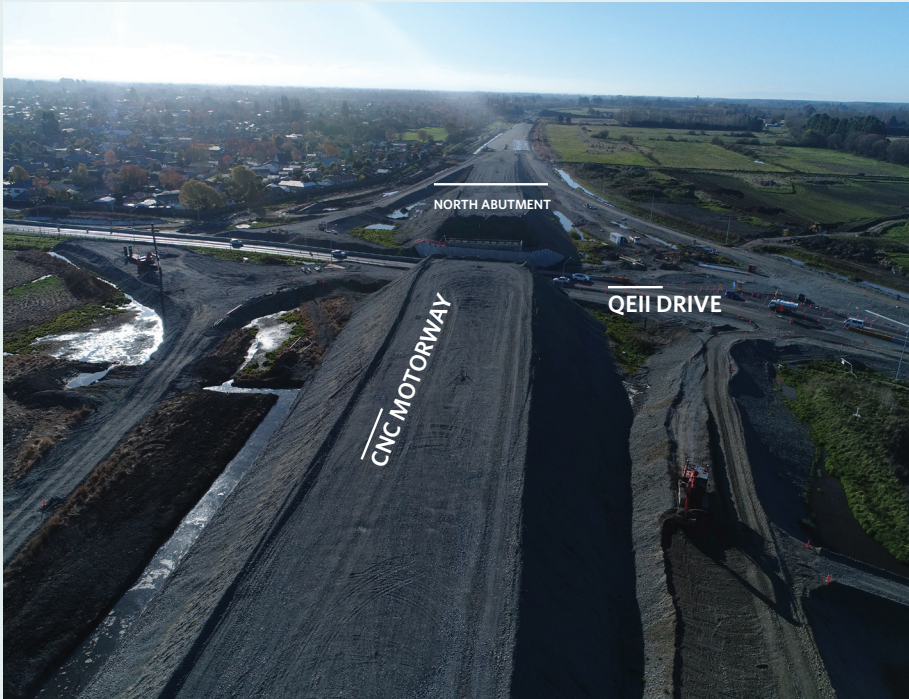
The new CNC motorway will go over QEII Drive while access to and from QEII Drive and the new motorway will be provided by double roundabouts below the bridge.
