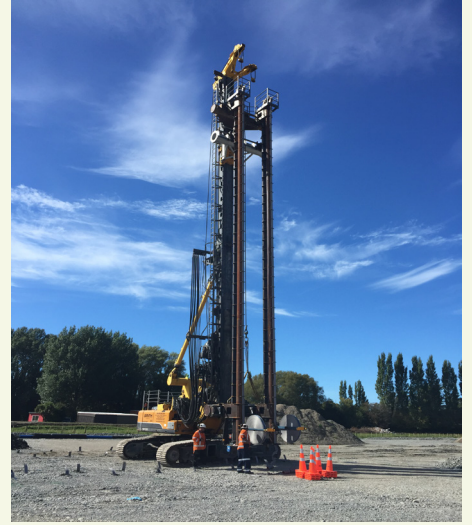
Left: Wick drains installed on alignment next to QEII Drive. Below: Twin mandrel rig used to install wick drains.
