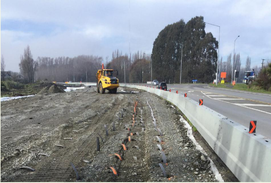
Left: Wick drains installed on alignment next to QEII Drive. Below: Twin mandrel rig used to install wick drains.
