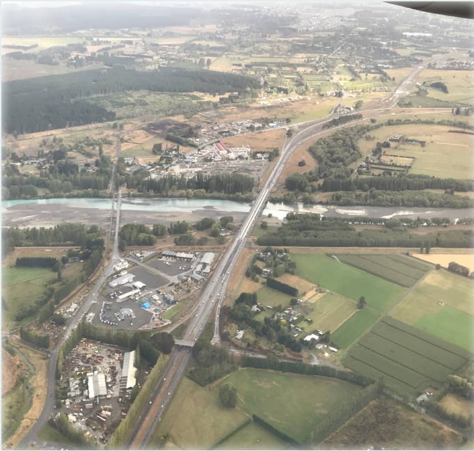
The project alignment looking south from Tram Road overbridge.
