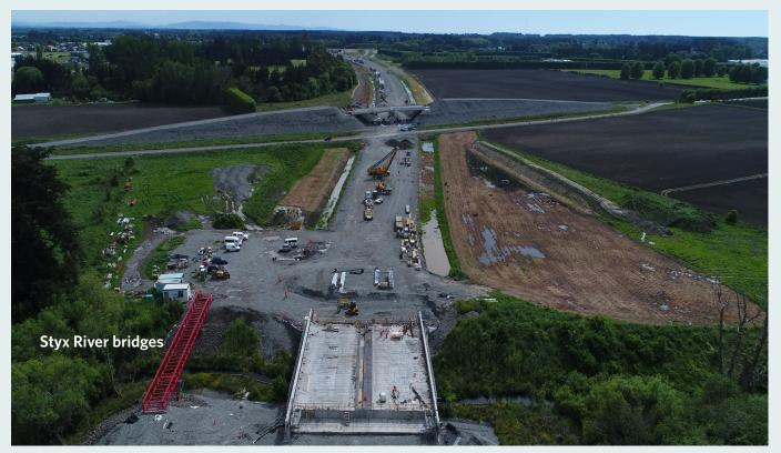
We recently lifted the deck into place for the separate pedestrian bridge over the Styx River(left in the photo). In the background is the Radcliffe Road bridge taking shape.
