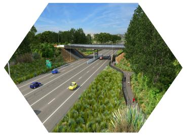
Prestons Road will pass over the top of the motorway on a bridge. Service lanes will be built for residents on the north side of Prestons Road. There will be no access to the motorway from Prestons Road. Pedestrian and cyclists can connect to the CNC shared use path along the motorway from Prestons Road.
