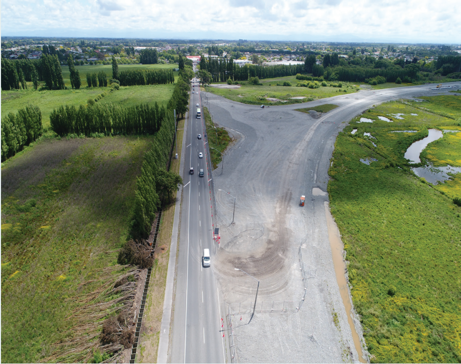
A roundabout will connect the motorway with Cranford Street.
