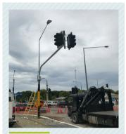
The new gantries will be put into the right positions over the road once the existing poles are removed.
