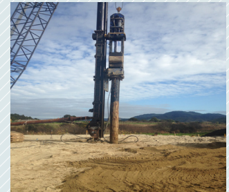
A similar timber piling rig in action
