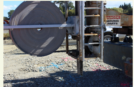
Image on the left: installation of wick drains using a twin mandrel rig. Image below: a closer look at the wick drain installation. Map below: the motorway work site area between Winters Road, QEII Drive and Prestons Road.
