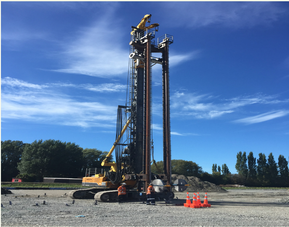
Image on the left: installation of wick drains using a twin mandrel rig. Image below: a closer look at the wick drain installation. Map below: the motorway work site area between Winters Road, QEII Drive and Prestons Road.
