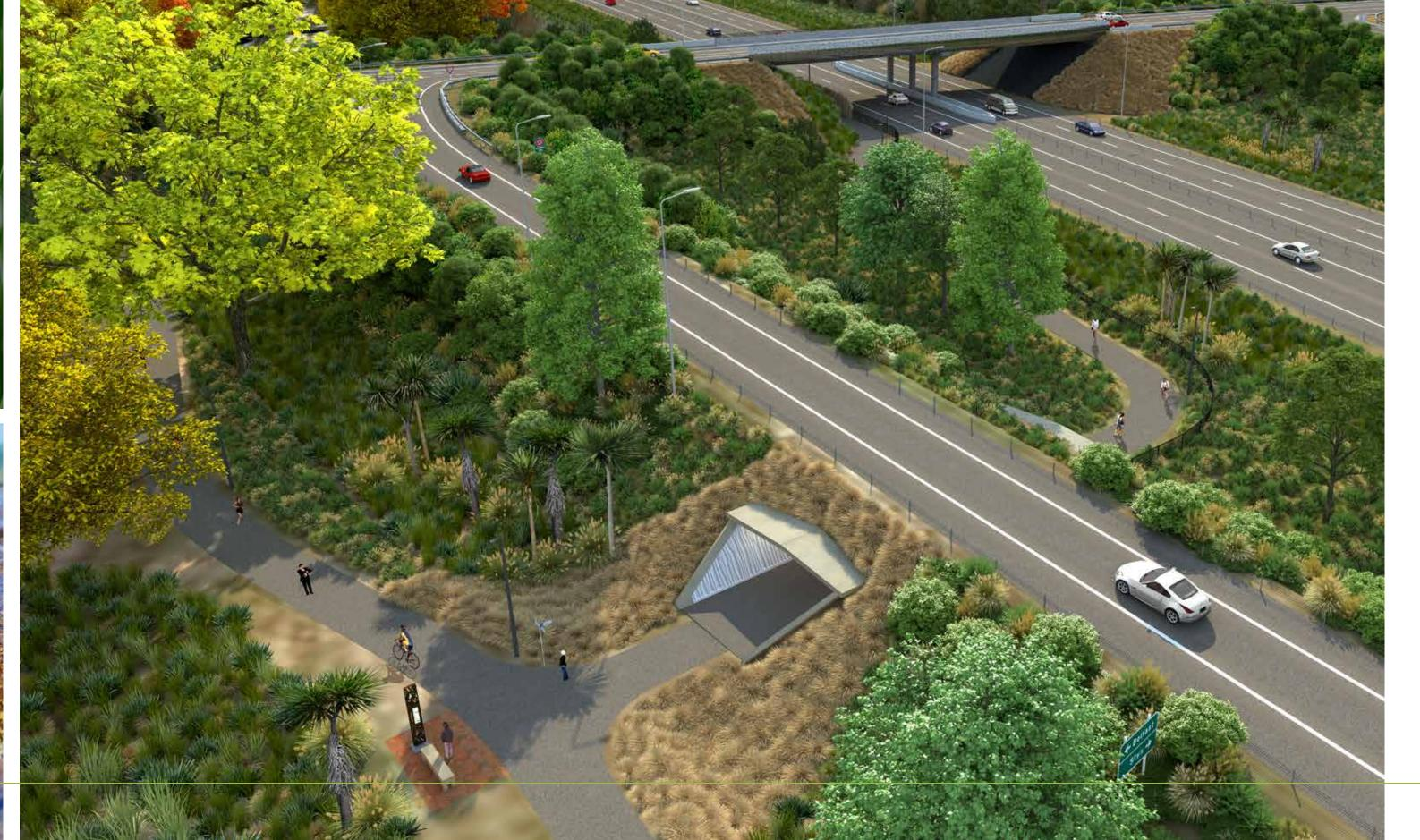
Guided by Sections 4.9 and 4.10 of the Agency's Urban Design Guidelines - Bridging the Gap, a key innovation of our urban design concept is the 'tilted walls' for new subways. This widened profile increases the sense of space and atmosphere for cyclists and pedestrians while adhering to low maintenance and easily constructive solutions. Key dimensions: tilted 30 degree wall profile. Internal subway height of 2.5m with a 5m wide floor.
